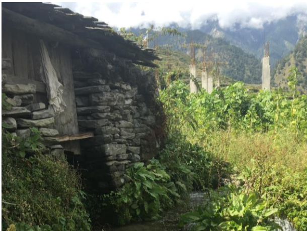
Figure 10. Downstream façade of a mill (Authors)
