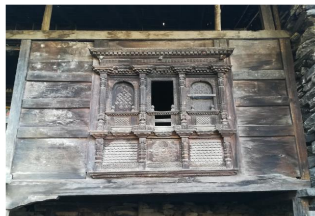
Figure 9. Wood facade (Authors)
